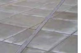
Concrete Pavers with Steel Inlay
