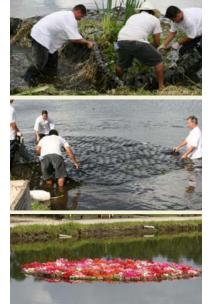
Beemats systems are designed for easy removal and recycling to maximize plant cleansing or reuse in a different way, such as this installation shown above
