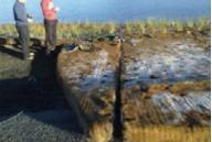
The wetland was constructed from over 400,000 plastic bottles (imported from the U.S.) topped with coconut fiber matting and over 20,000 native plants. Modules were bolted together with steel and wire (like knitting a scarf row by row).
